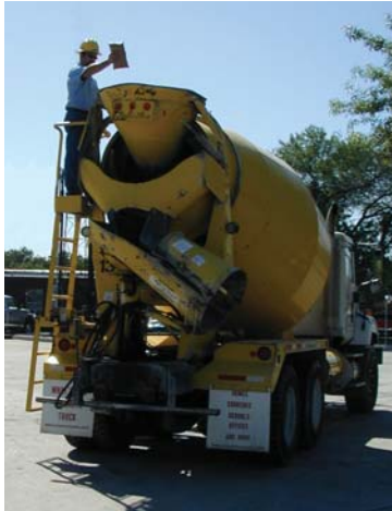
Add Fritz-Pak products directly into the ready mix truck
